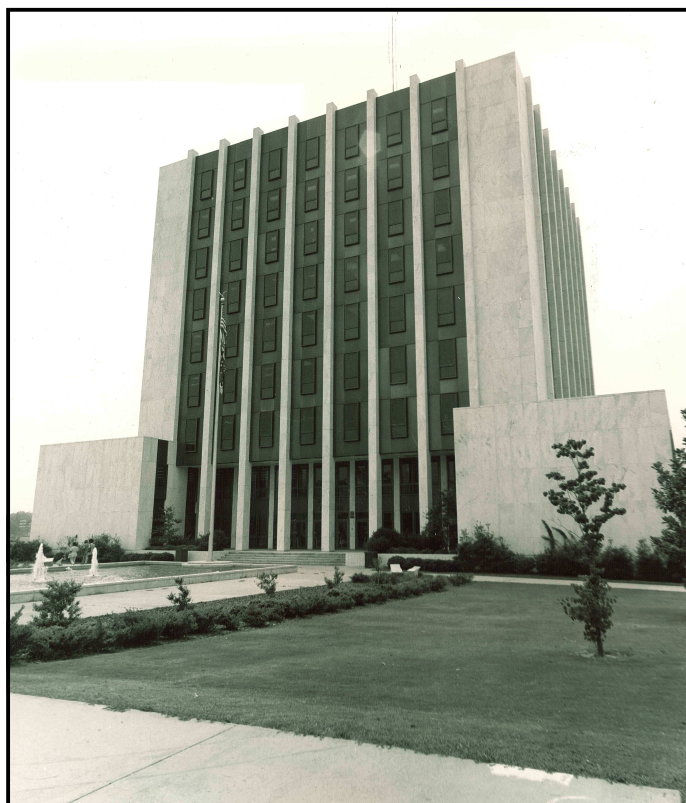
The DeKalb County Courthouse is located at 556 N. McDonough Street, Decatur GA 30030.
